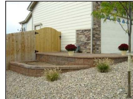
The Cuesta Cap is split on both the front and the back sides. This allows installers to flip-flop the caps in straight walls and create a
