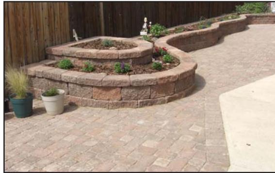
There are three gravity wall systems: core-fill, lip and pin. Our Cuesta System is core-fill, which means structural integrity is obtained by filling the large voids in each block with crushed rock. The aggregate forms stabilized columns that span from bottom to top, locking the wall together. Crushed rock is required by every retaining wall system, allowing water to drain rapidly through the wall to avoid failure. *Please review the installation instructions.*
