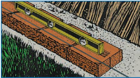
Place the first layer of Pyzique stones **smooth side down** on the prepared foundation. Use a level in all directions and use a string line to verify straightness. Serpentine walls may be built. Be certain the base course is level and stones lay flat. For micro leveling and to help the stones lay flat use small handfuls of sand to level and stabilize the first course.
