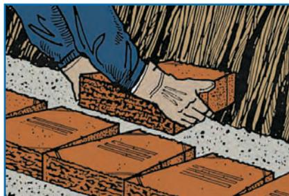
The normal bottom of each Pyzique stone is smooth. Place the **bottom up** for your cap layer. To avoid vandalism, use a **paver grade glue** to secure the cap layer to the layer below it. The cap layer may be set 1" forward for a cap layer overhang.
