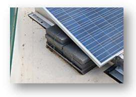
High compressive strength and density combined with low absorption are important to the long-term durability of the concrete. Lower-quality concrete can deteriorate in under a decade due to the aggressive freeze/thaw environment that the roofs and the ballasts create.
